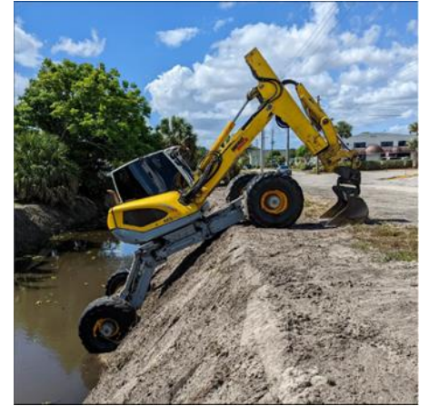
Menzi Truck for ditch cleaning
