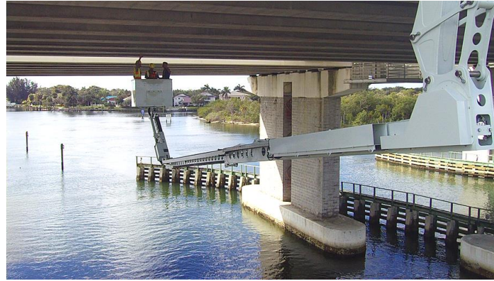
Under bridge bucket truck for bridge maintenance
