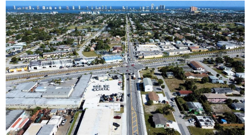
Silver Road Project Overseen by Construction Coordination
