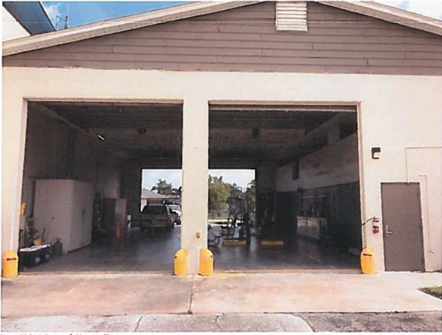
East Side View of City Hall
