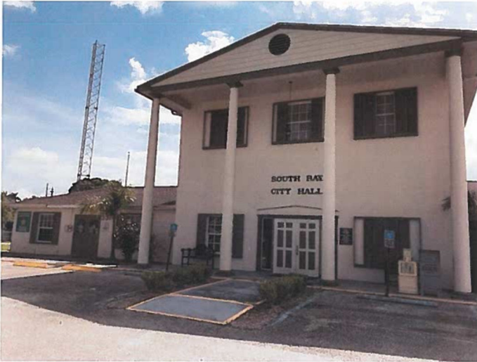
Front Facing West View of City Hall Chambers and Public Safety Office
