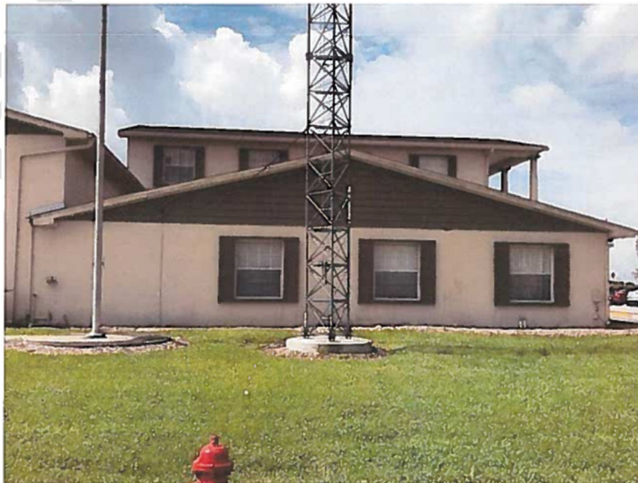
North East Side View of City Hall
