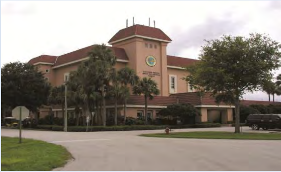
Southern Regional Water Reclamation Facility
