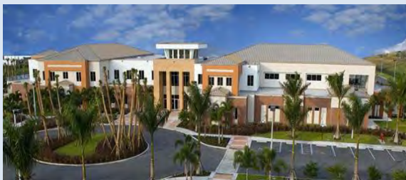
Fire Rescue Headquarters
