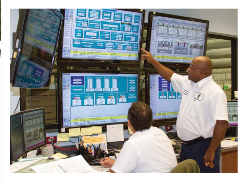
Water plant operators Water Treatment Plant 9 Boca Raton, FL
