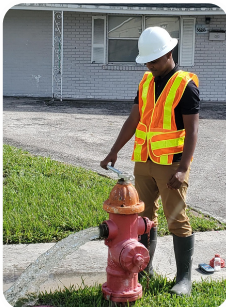
YEC Summer Internship - student interning with the City of Riviera Beach Water Utility Department flushing the fire hydrant
