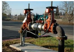
Backflow prevention devices are used to prevent contaminated fluids or gases from entering into a potable water supply system and are required at all premises likely to have cross-connections as part of the Town's cross-connection control program. "Cross-connections are the links through which it is possible for contaminating materials to enter into a potable water supply through backflow."<sup>5</sup>
